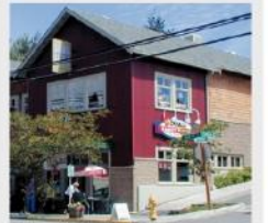
Figure 6-41. This building uses an acceptable combination of metal siding, concrete block and wood shingles (Duvall, WA).
