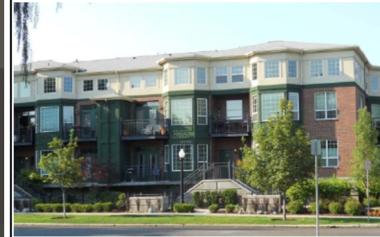
Fig. 4-30. Examples of windows that are recessed from the facade by at least two inches. Notice how this creates shadows on the windows, which lends depth and interest to the facade.
