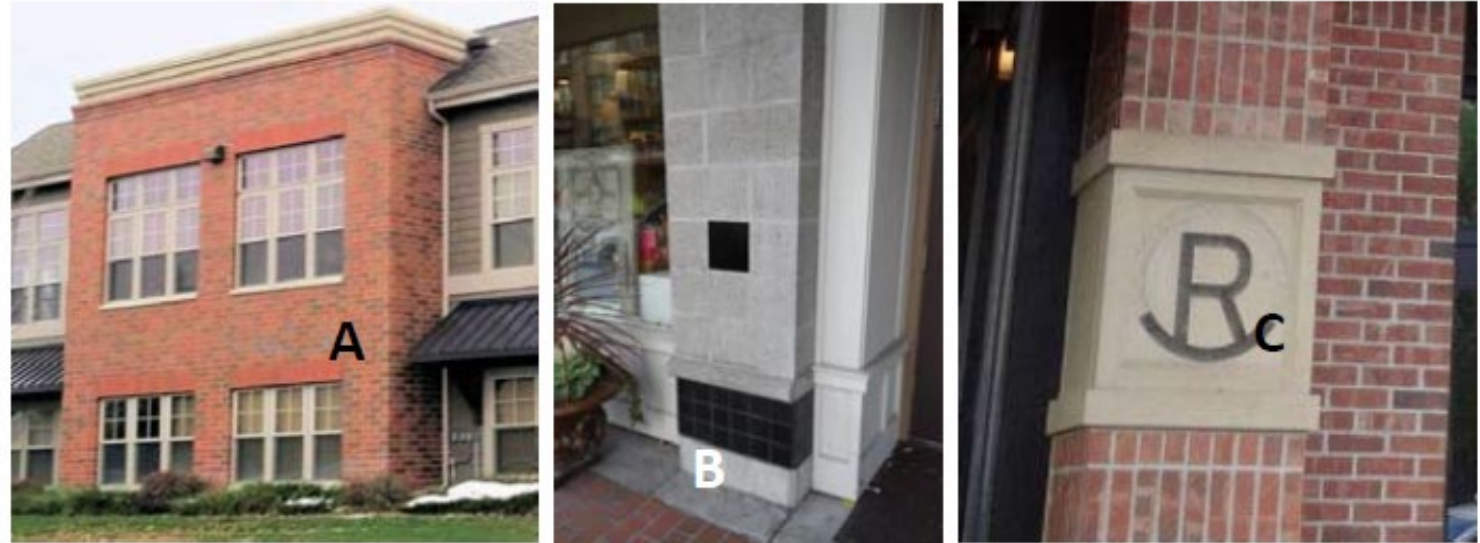
Examples of decorative surface materials. A = decorative brick/design. B = decorative tile-work and column pattern. C = decorative medallion.
