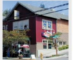
Figure 6-41. This building uses an acceptable combination of metal siding, concrete block and wood shingles (Duvall, WA).
