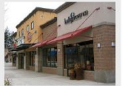
Figure 6-44. This building combines stucco and concrete block.
