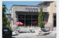
Figure 6-43. This building employs a single type of concrete block, but it comprises less than 50% of the façade (Snoqualmie, WA).
