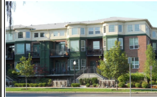
Fig. 4-30. Examples of windows that are recessed from the facade by at least two inches. Notice how this creates shadows on the windows, which lends depth and interest to the facade.
