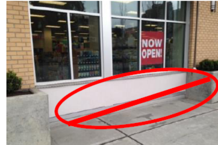
Figure 20.131.060.C.3 Acceptable and unacceptable EIFS examples.
