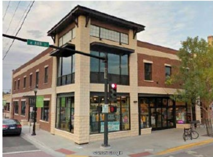
Figure 20.131.060.C.1 Acceptable concrete block use/design.
